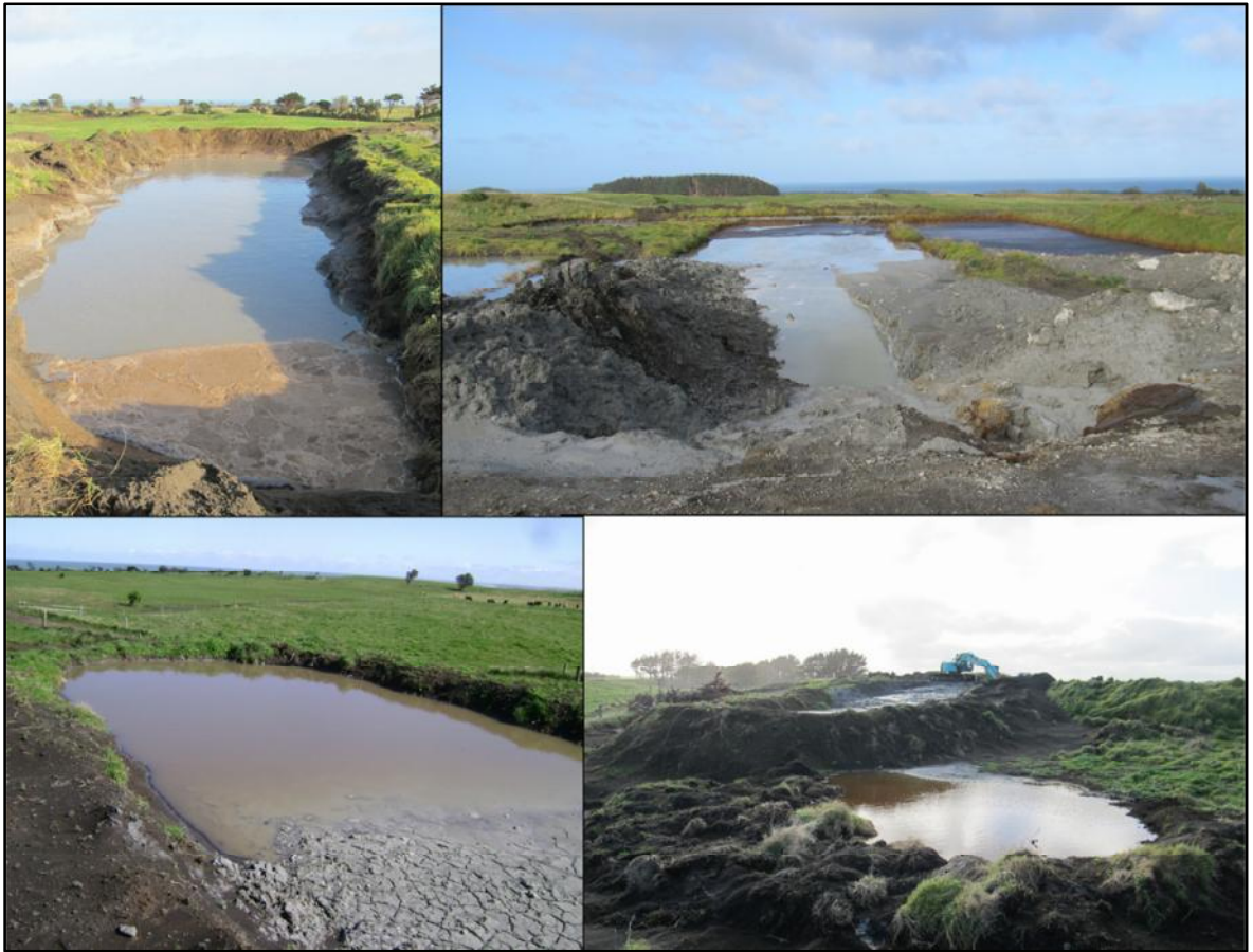
Figure 4 Photographs of waste stored poorly in unlined pits at Waikaikai landfarm under Redback management
