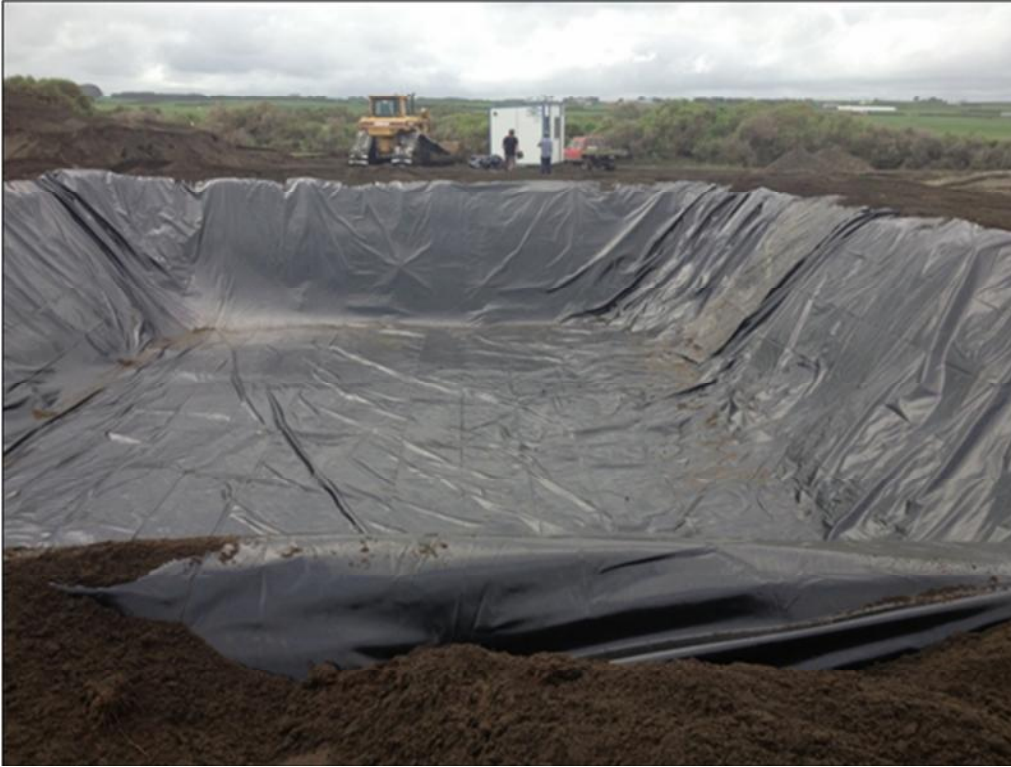
Photo 2 Pit-C newly constructed showing high grade HDPE synthetic liner
