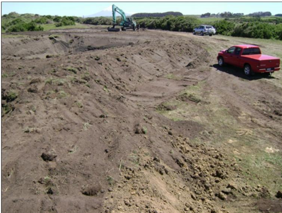
Photo 1 Initial earthworks at Vanner landfarm showing stockpiling area construction
