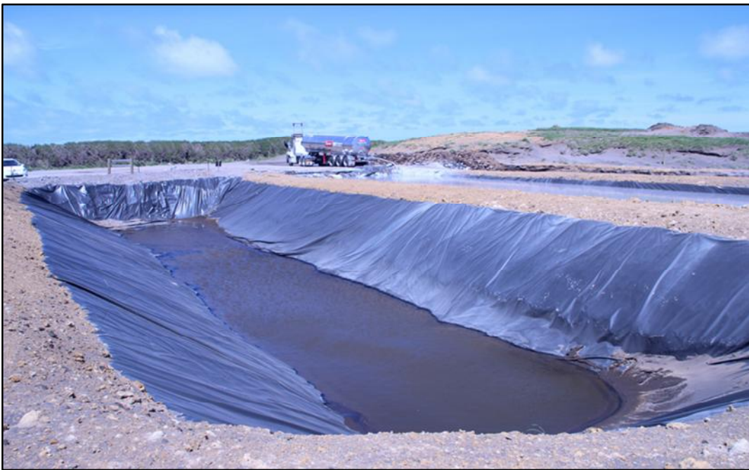
Photo 3 Oeo landfarm pits showing HDPE synthetic liners
