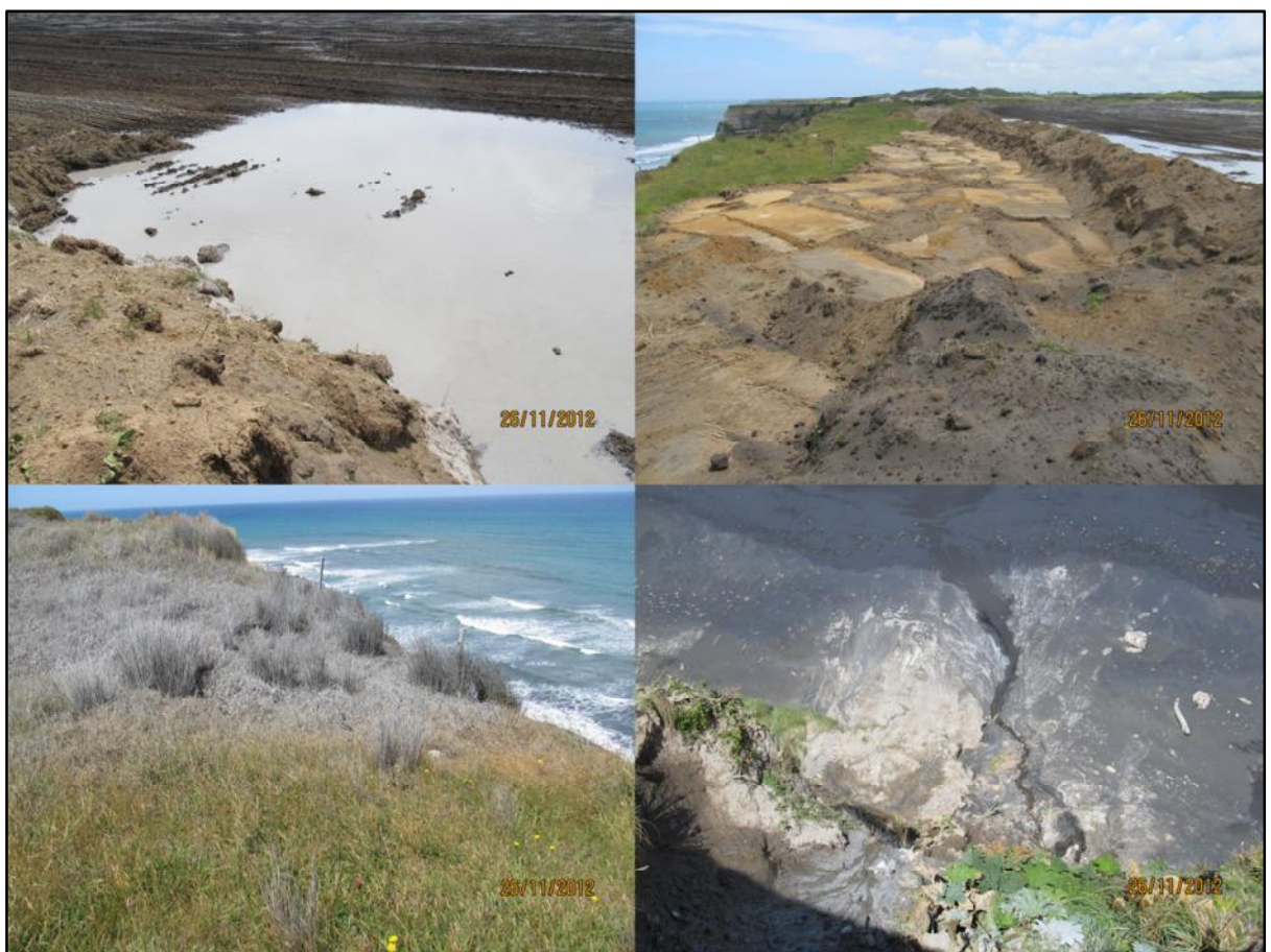
Figure 4 Oeo landfarm photos showing (clockwise from top left) ponding liquid in area F2, makeshift bunding in buffer zone, mud on beach below cliff, and mud staining of grass
