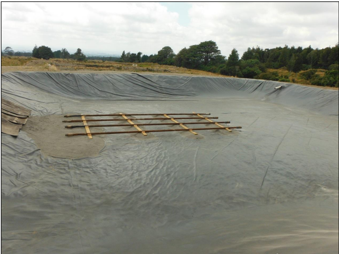
Photo 5 Newly lined pits at Surrey Road stockpiling facilities
