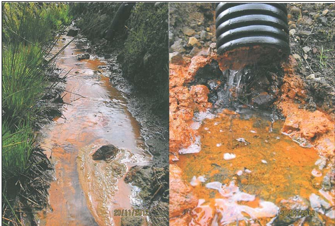
Photo 4 Periphery drain, Surrey Road stockpiling looking upstream to perforated pipe 1 (left) and water discharging from perforated pipe 2 (right)
