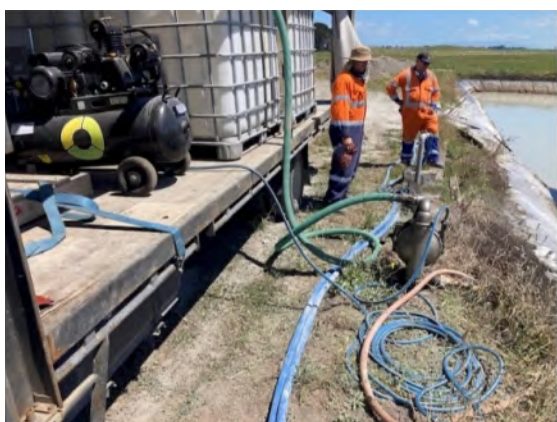
Photograph 3: Removal of oil slick by air diaphragm vacuum pump
