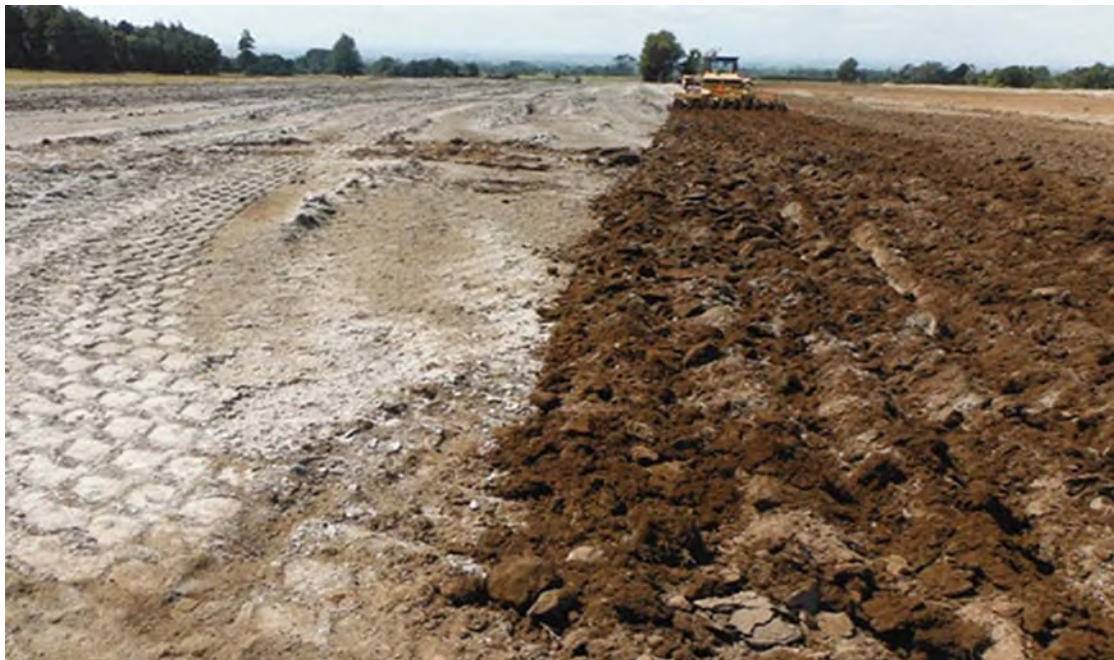
Photo 2 Drilling waste being tilled into the soil
