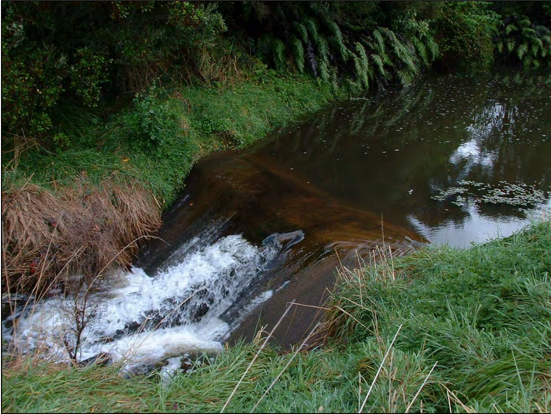
Photo 1 McKee Production Station water supply weir in Mangahewa Stream, with the fish pass in the centre of the weir.
