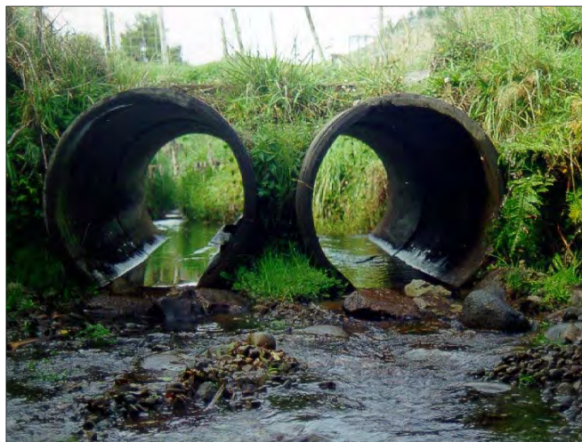
Photo 2 Farm access crossing, located in the Mangahewa Stream just downstream of the McKee Production Station water supply weir.
