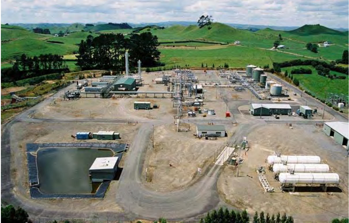
Photo 1 Waihapa Production Station
