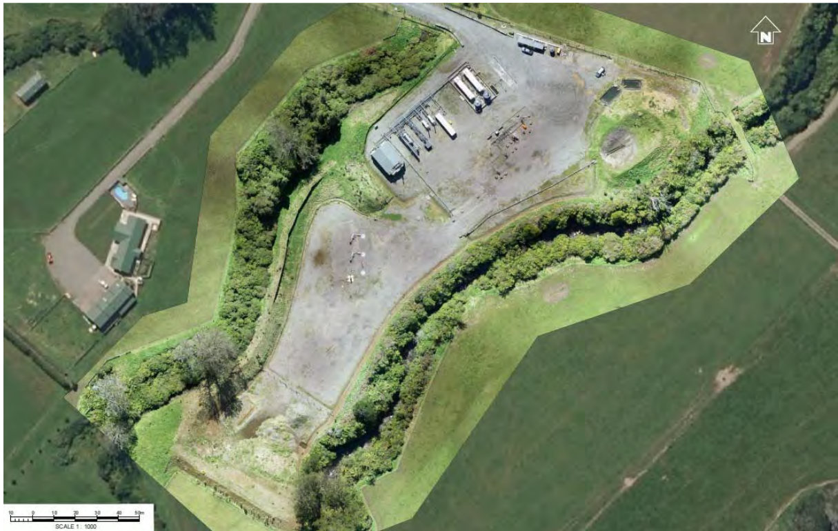
Photo 1 Sidewinder Production Station and wellsite in 2017
