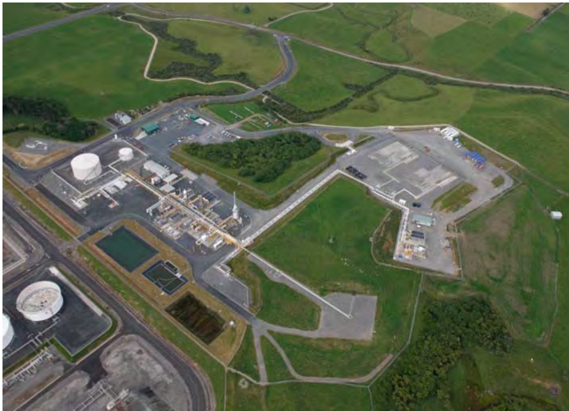
Photo 3 Pohokura Production Station
