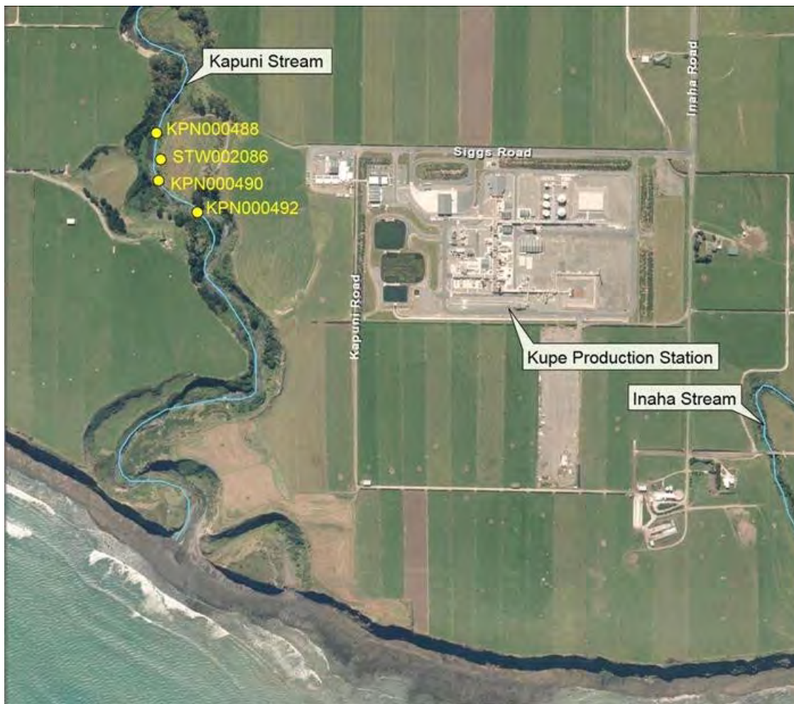
Figure 4 Location of the Kupe Production Station and associated monitoring sites
