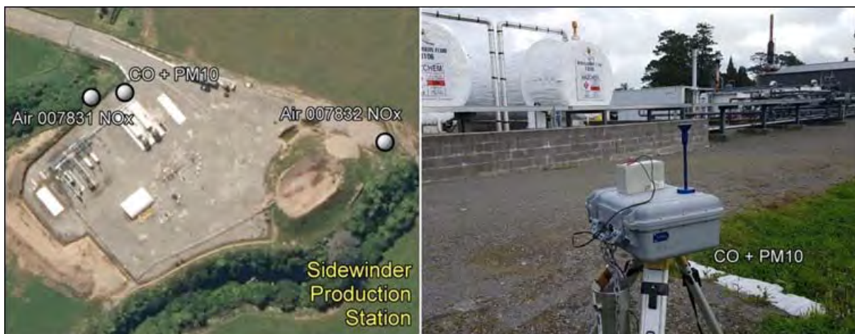
Figure 2 Air monitoring sites at Sidewinder Production Station for 2016-2017
