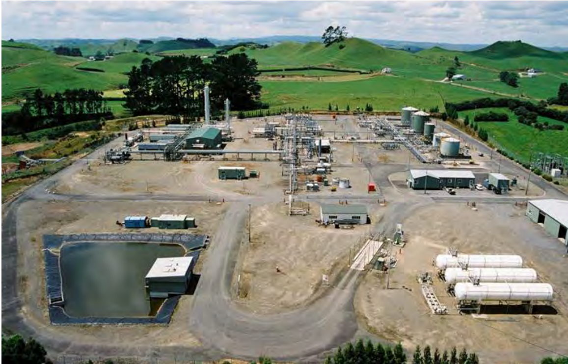
Photo 1 Waihapa Production Station
