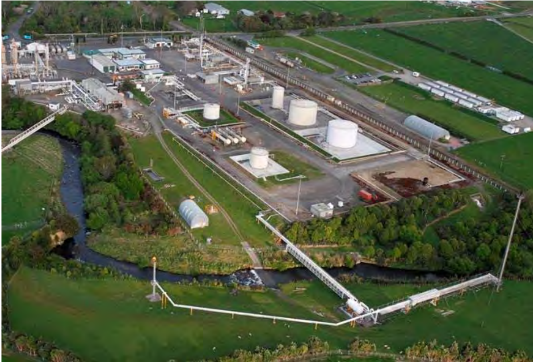
Photo 1 Kapuni Production Station
