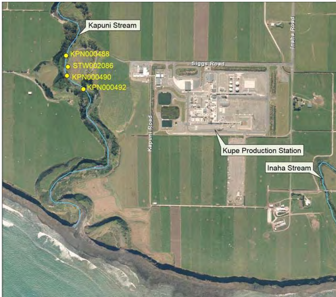
Figure 3 Location of the Kupe Production Station and associated monitoring sites
