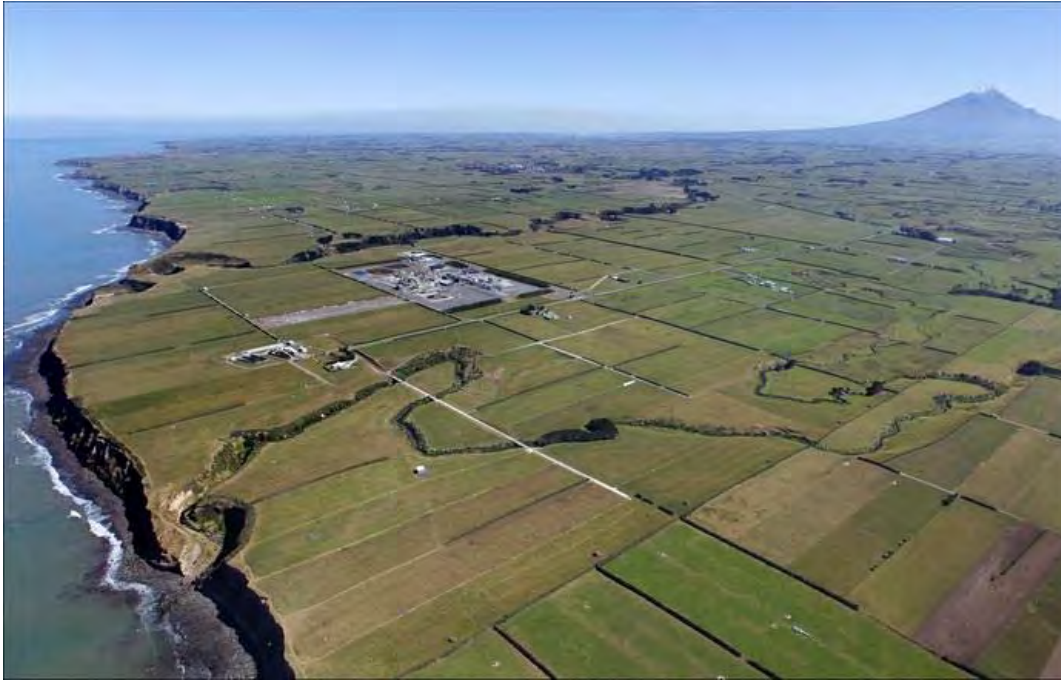
Photo 1 Kupe Production Station
