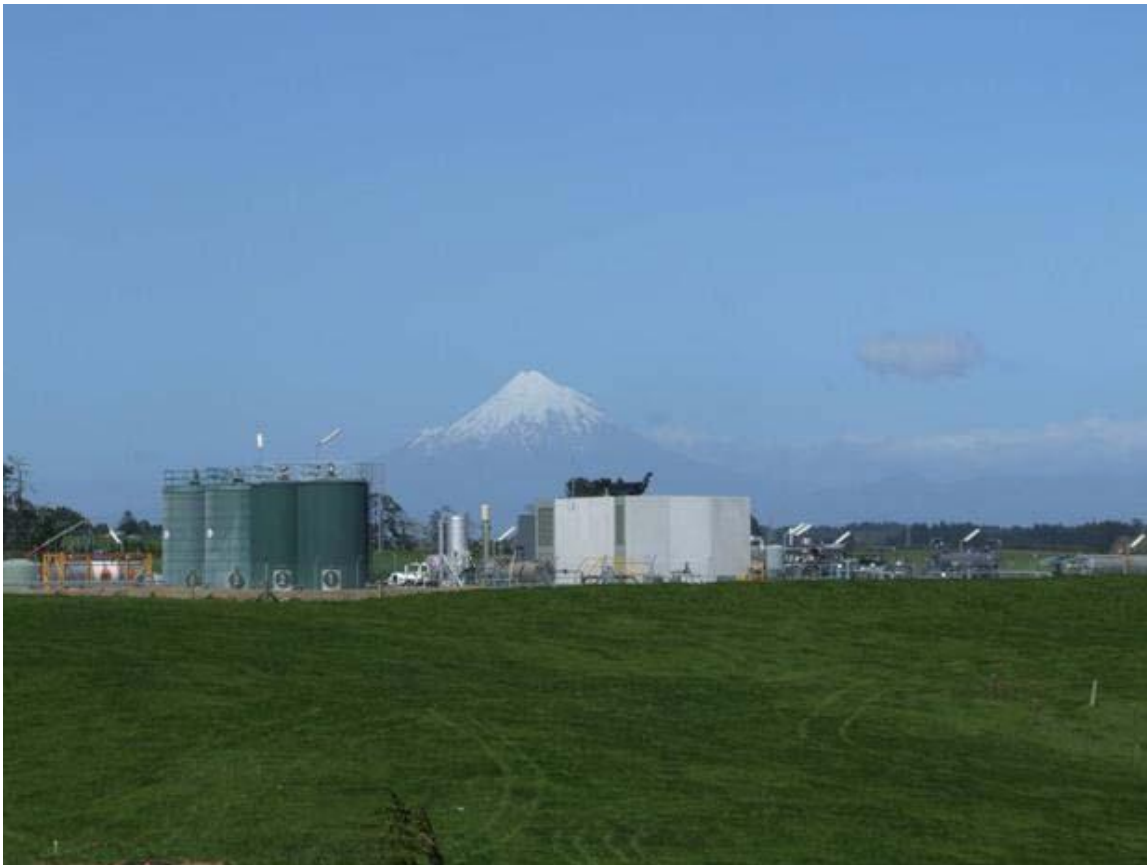
Photo 1 Turangi Production Station
