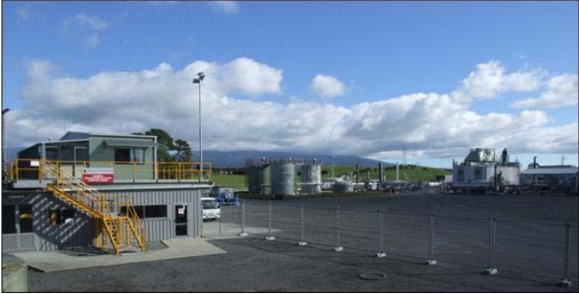
Photo 1 Kaimiro Production Station
