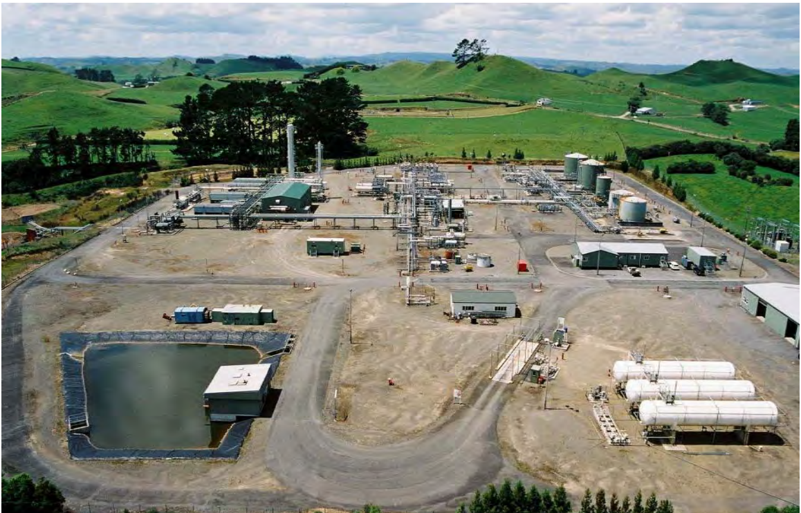
Photo 1 Waihapa Production Station
