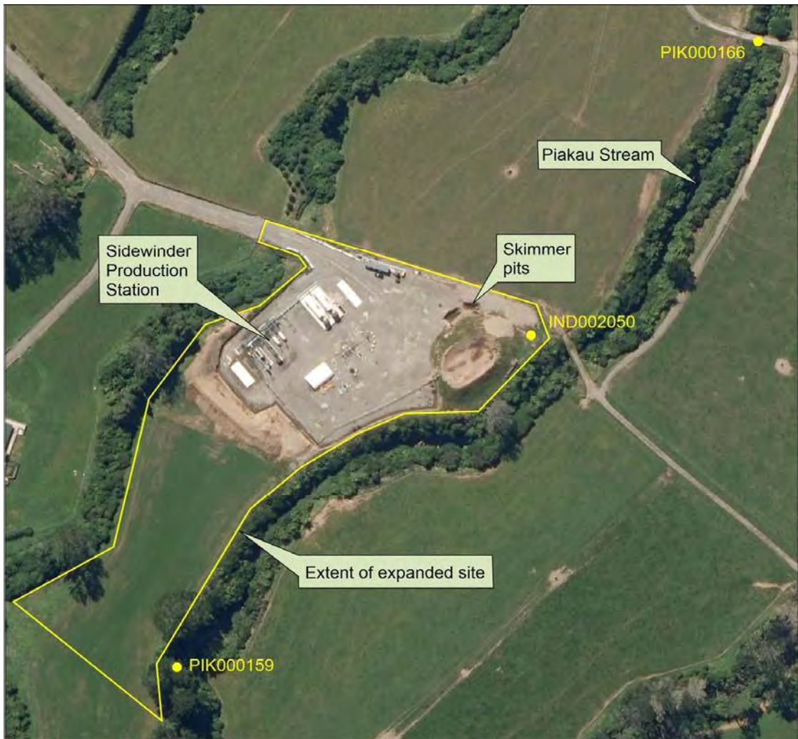
Figure 1 Sidewinder Production Station and associated water quality sampling sites
