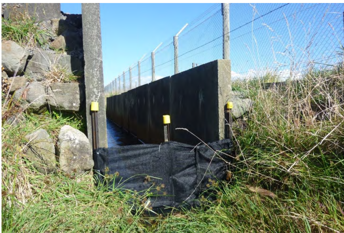
Photo 2 Silt cloth installed in a perimeter stormwater drain at the Maui Production Station, April 2013
