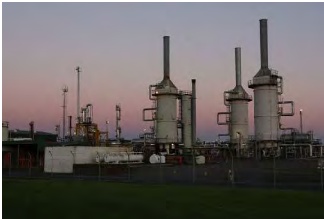
Photo 3 Emissions sources at the Maui Production Station
