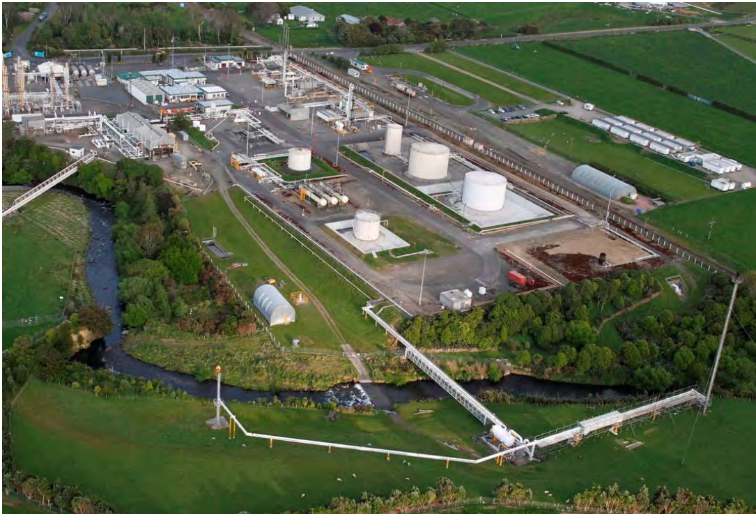
Photo 1 Kapuni Production Station
