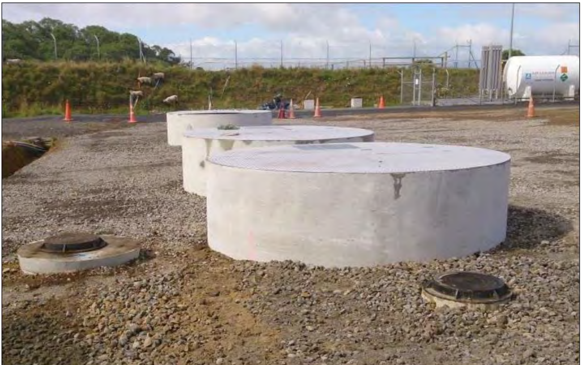
Photo 2 Upgraded stormwater system at the Lower Otaraoa Road wellsite
