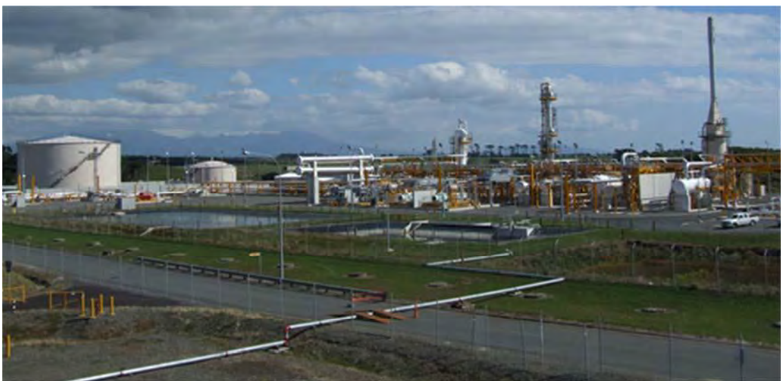
Photo 1 Pohokura Production Station
