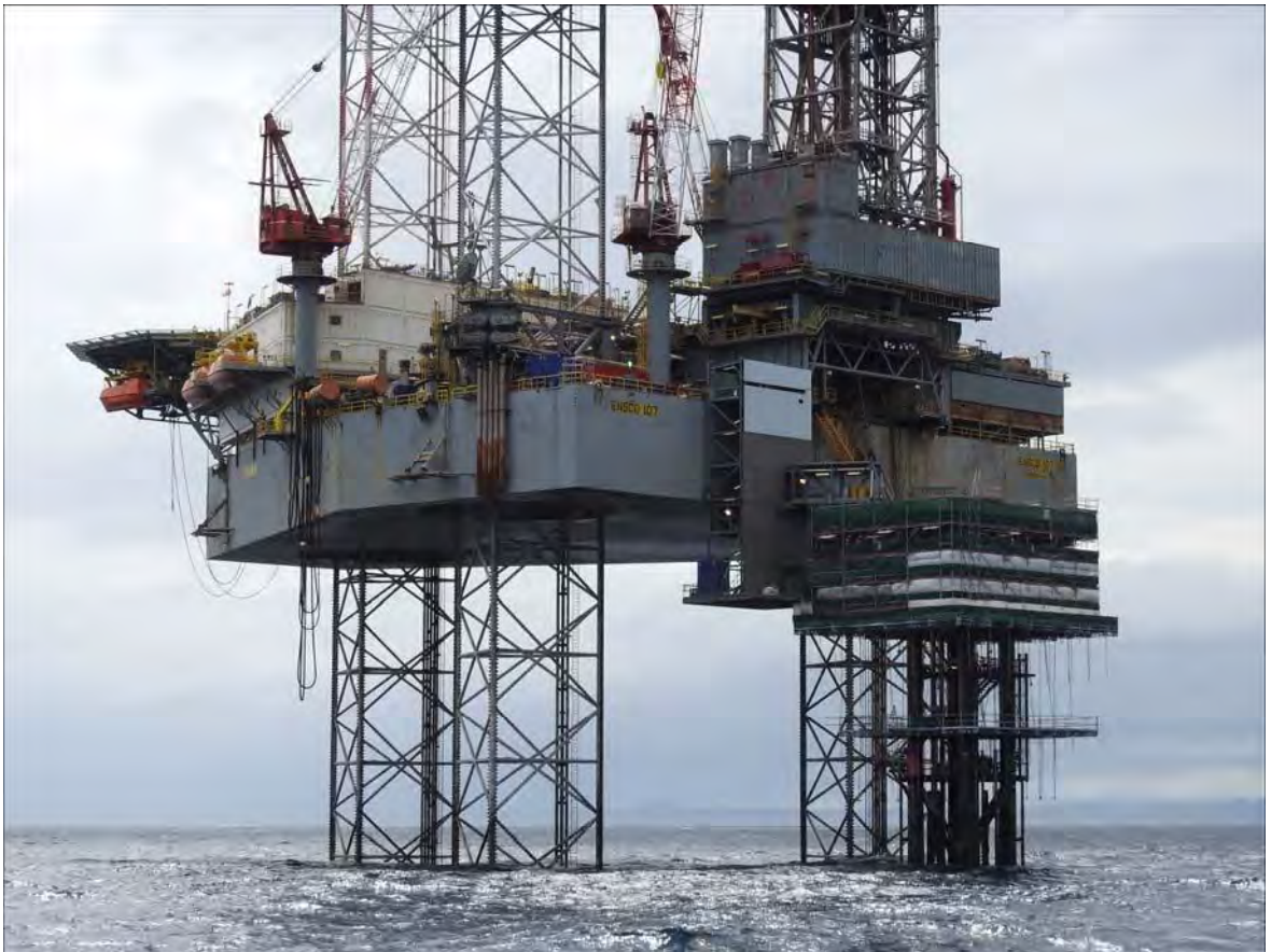
Photo 3 The EnSCO 107 jack-up rig adjacent to the Pohokura Platform B during refurbishment works
