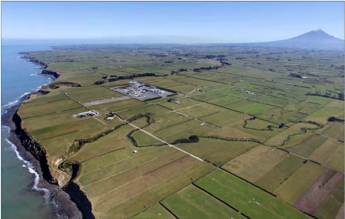
Photo 1 Kupe Production Station
