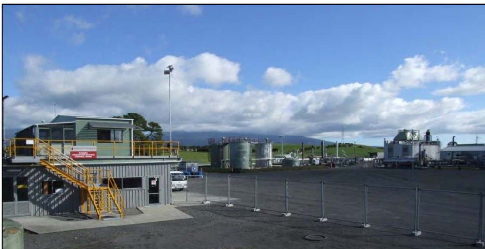
Photo 1 Kaimiro Production Station
