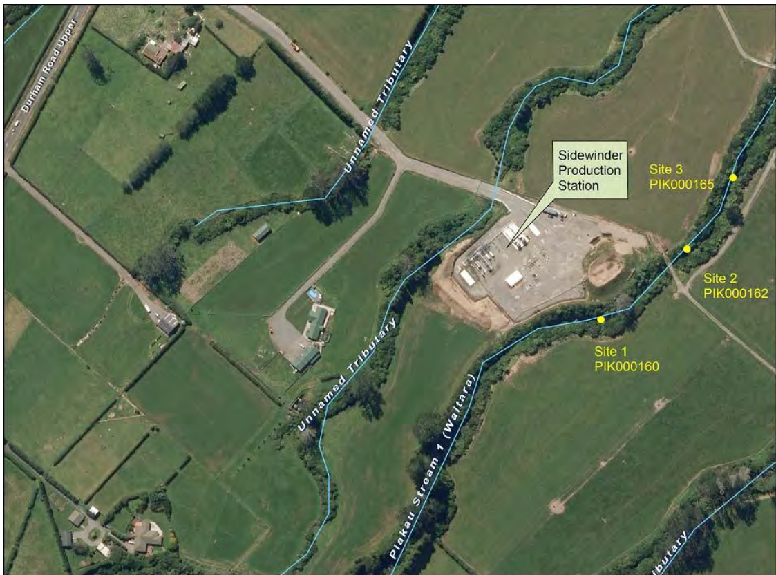
Figure 2 Biomonitoring sites in the Piakau Stream adjacent to the Sidewinder Production Station
