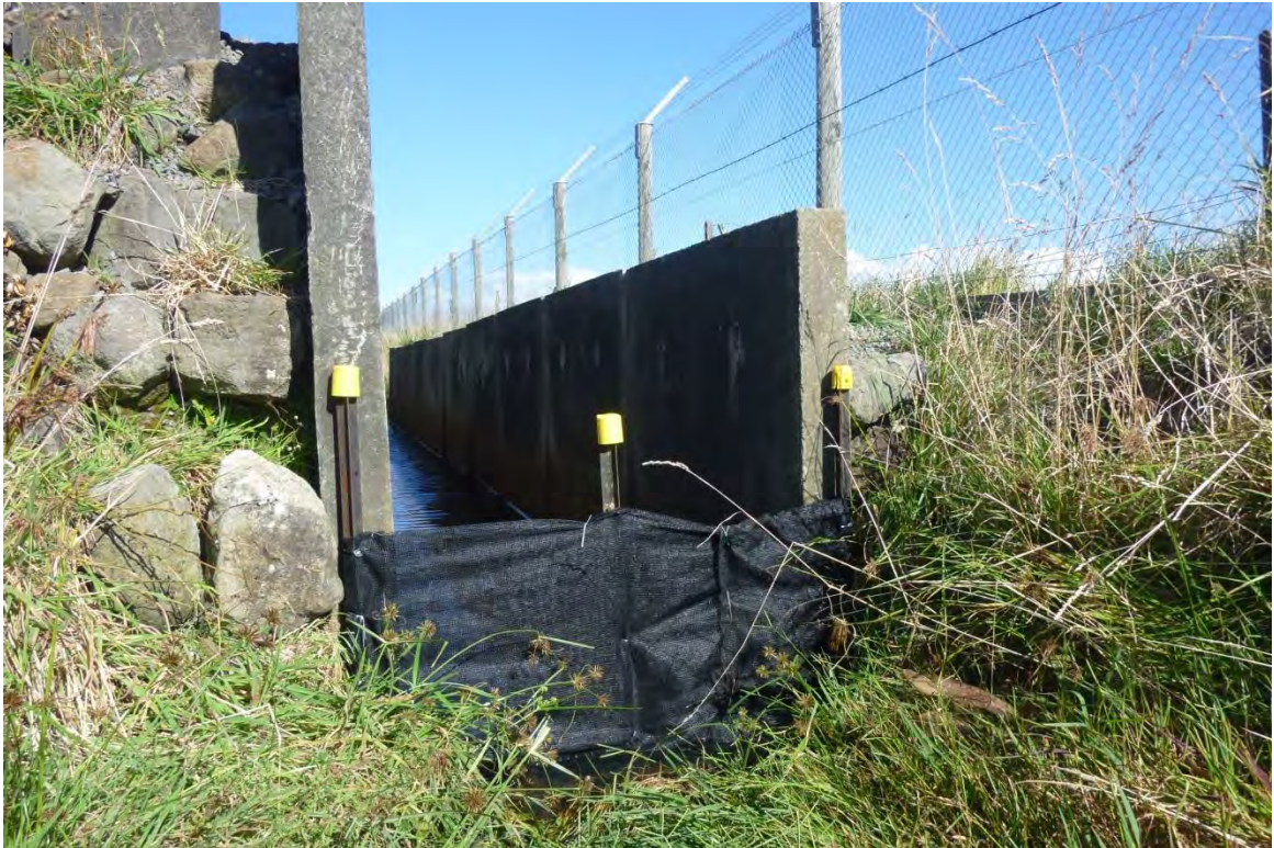
Photo 2 Silt cloth installed in a perimeter stormwater drain at the Maui Production Station, April 2013
