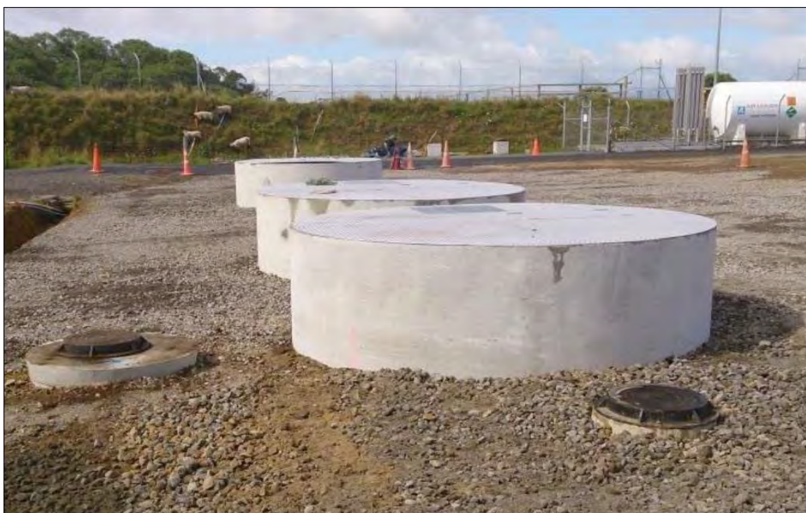
Photo 2 Upgraded stormwater system at the Lower Otaraoa Rd wellsite
