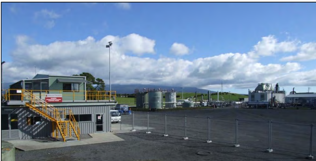
Photo 1 Kaimiro Production Station
