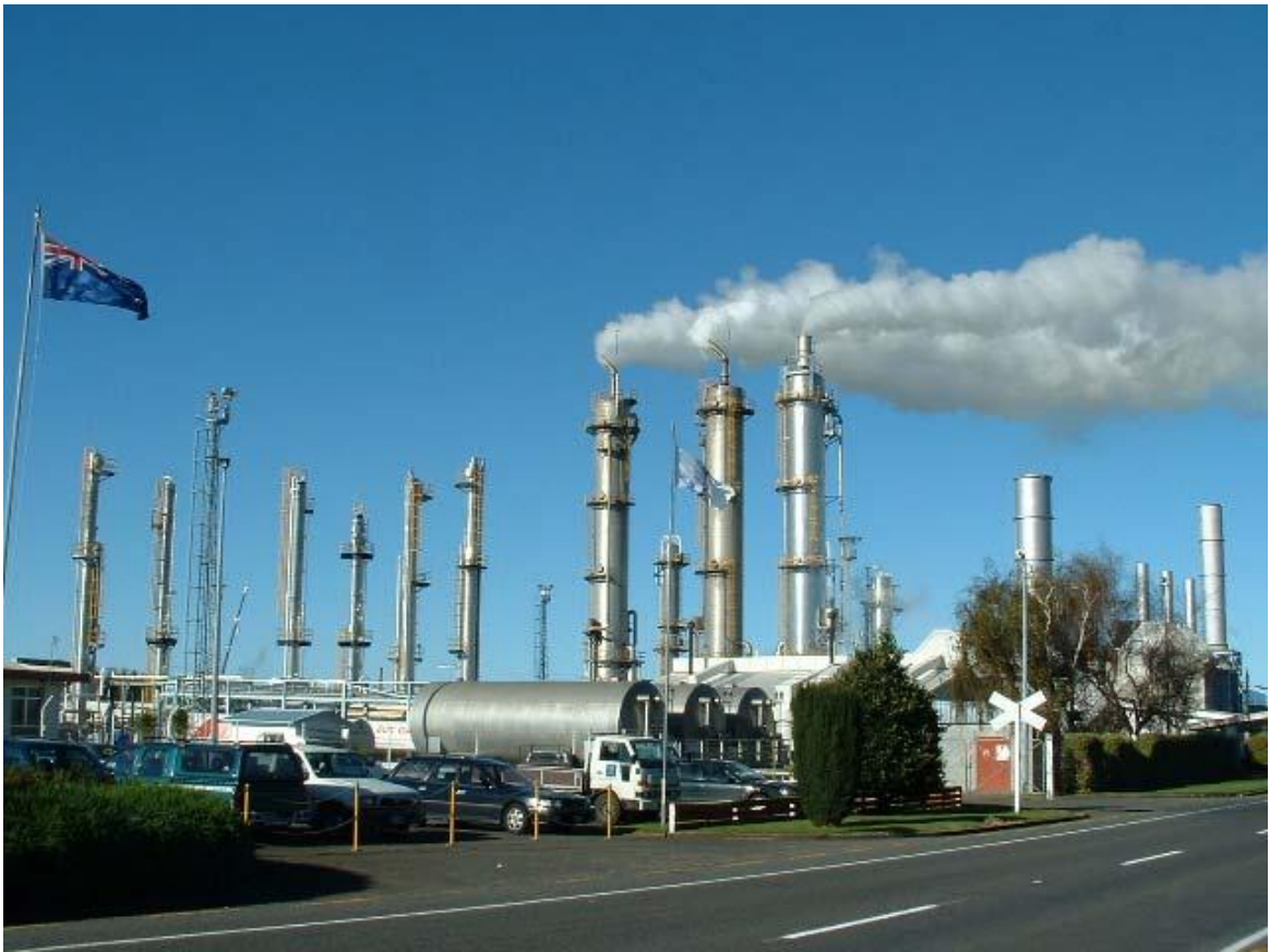
Photo 1 Vector Kapuni gas treatment plant during three-train operation
