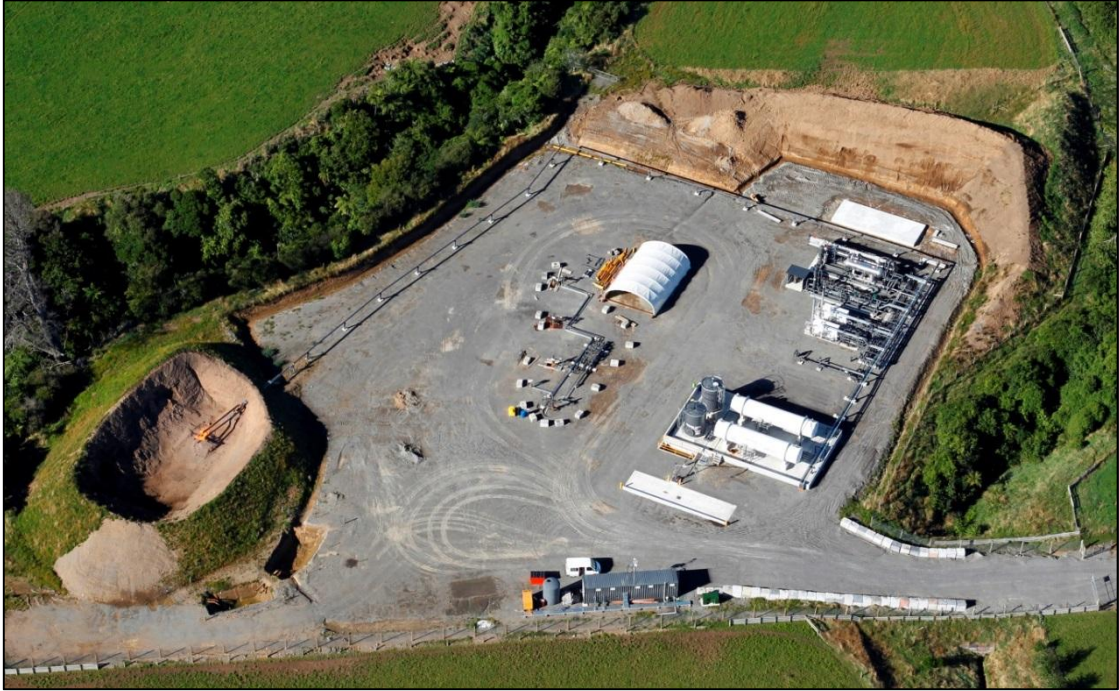
Photo 1 Sidewinder Production Station and wellsite in February 2012
