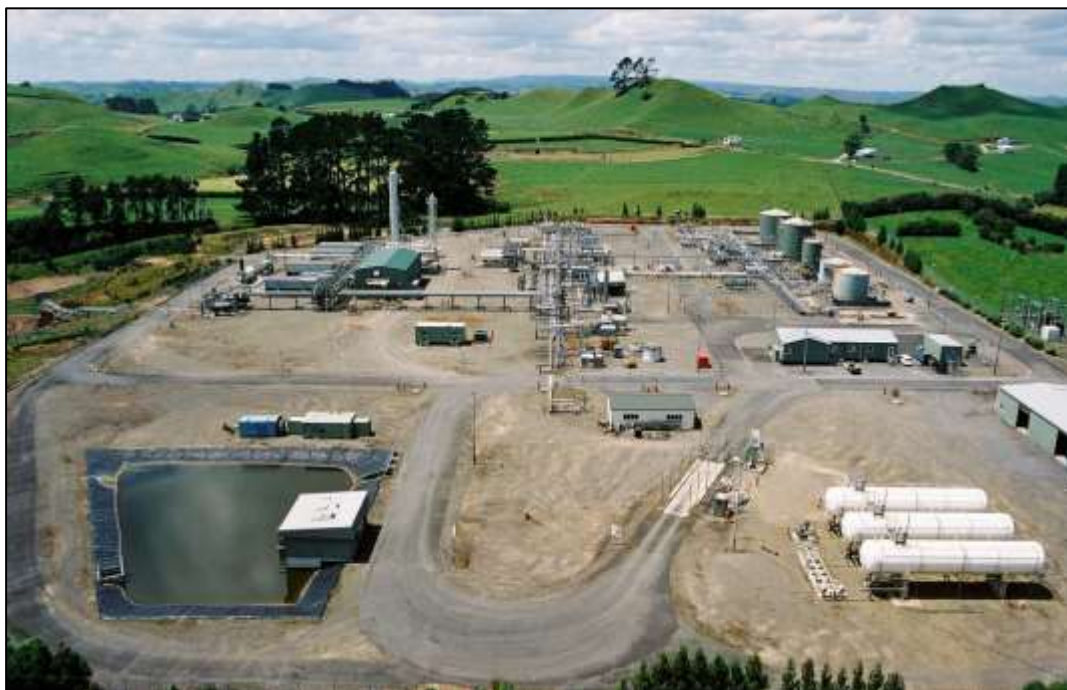
Photo 1 Waihapa Production Station
