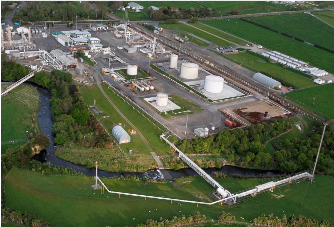
Photo 4 Kapuni Production Station
