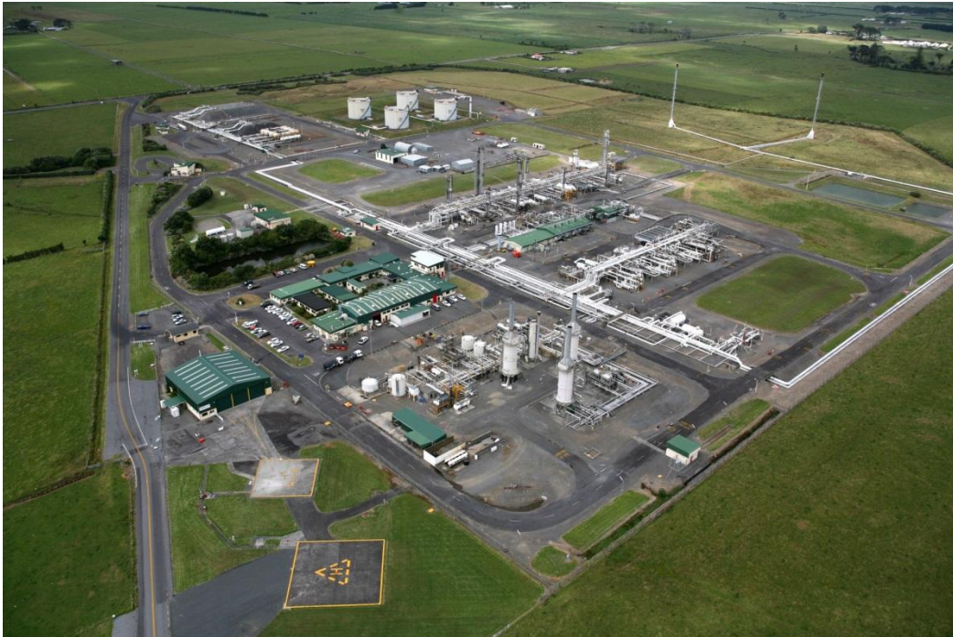
Photo 1 Maui Production Station
