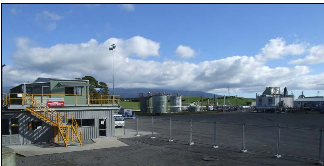
Photo 1 Kaimiro Production Station
