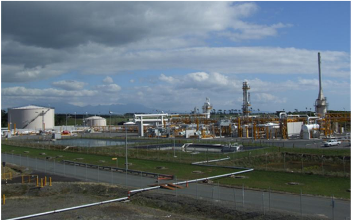
Photo 1 Pohokura Production Station
