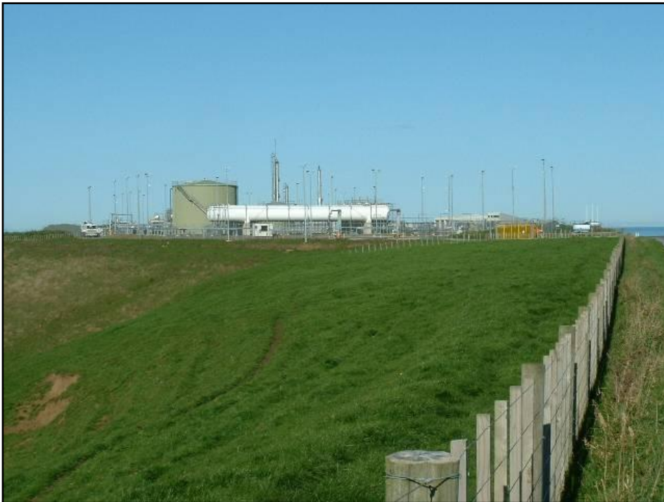
Photo 1 Rimu Production Station
