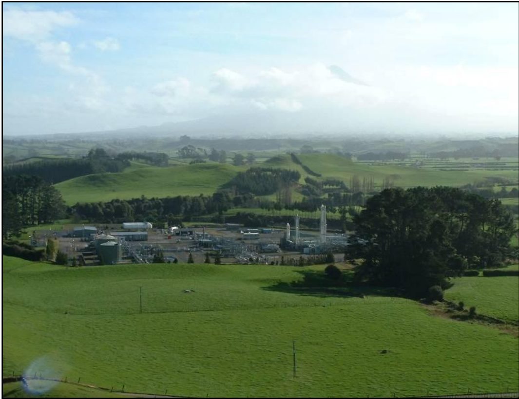
Photo 2 Waihapa Production Station
