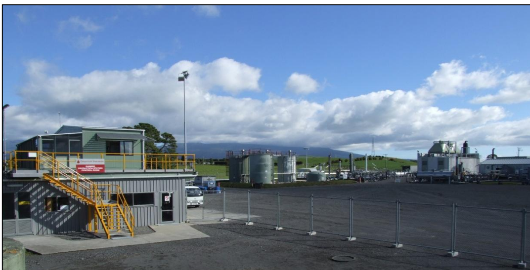
Photo 1 Kaimiro Production Station
