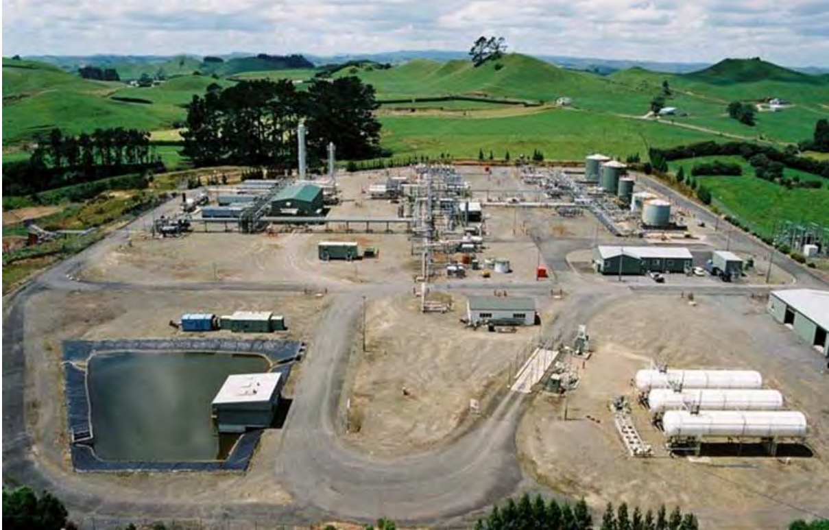
Photo 1 Waihapa Production Station
