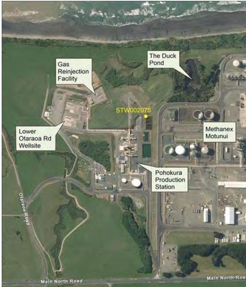
Figure 1 Pohokura onshore facilities and the combined discharge sampling site STW002075
