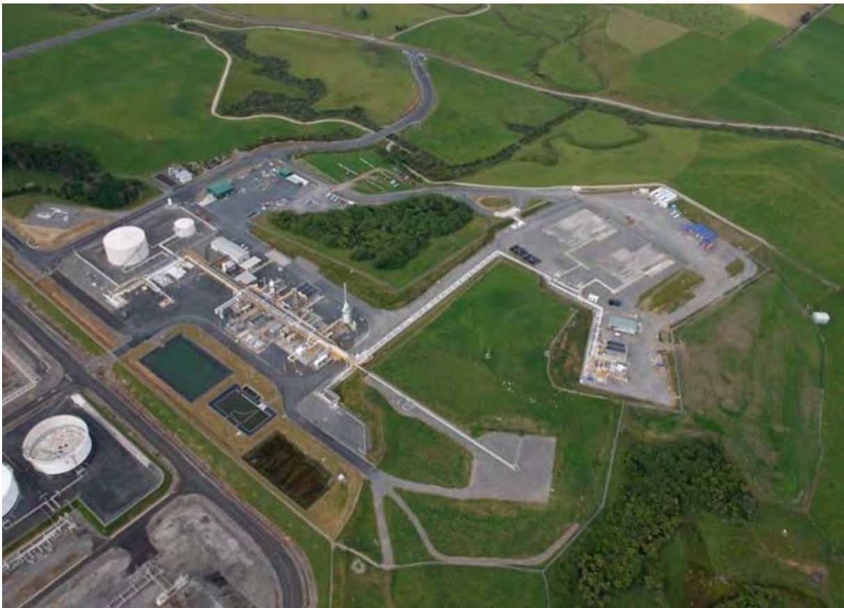
Photo 3 Pohokura Production Station
