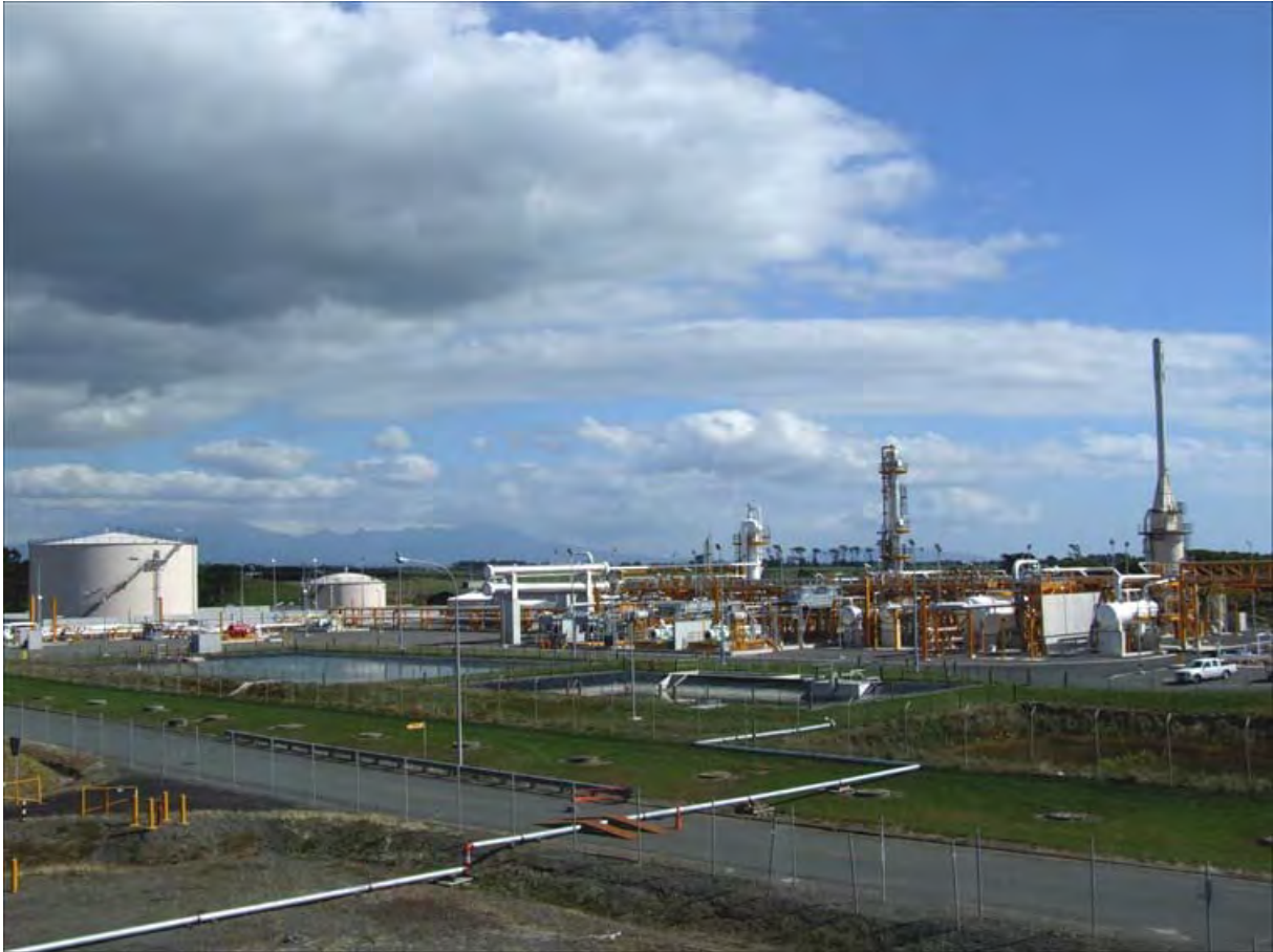
Photo 1 Pohokura Production Station
