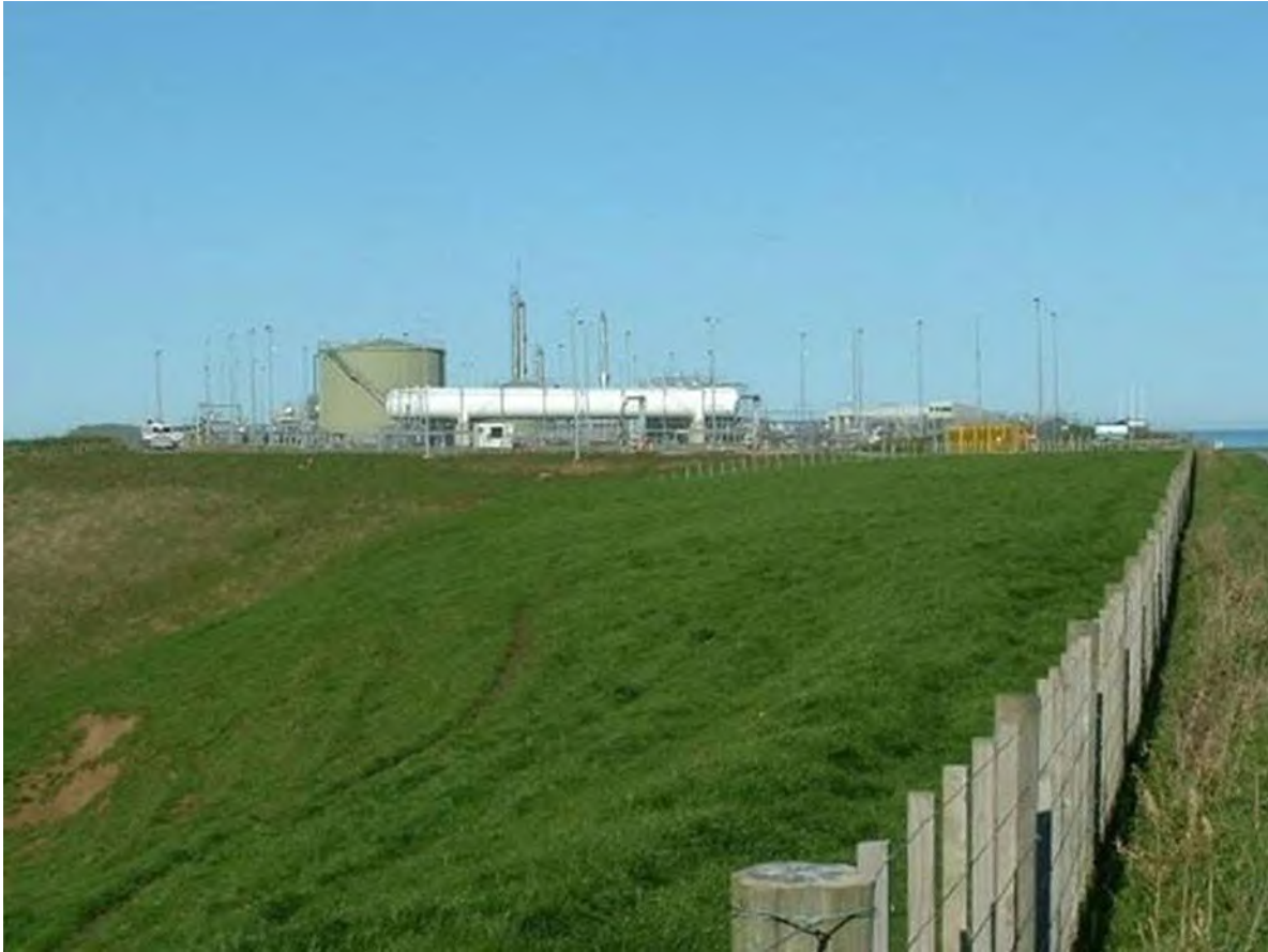
Photo 1 Rimu Production Station
