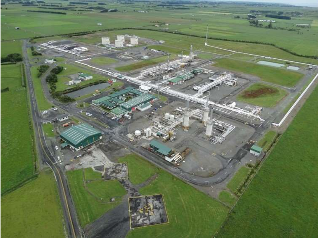
Photo 1 Maui Production Station
