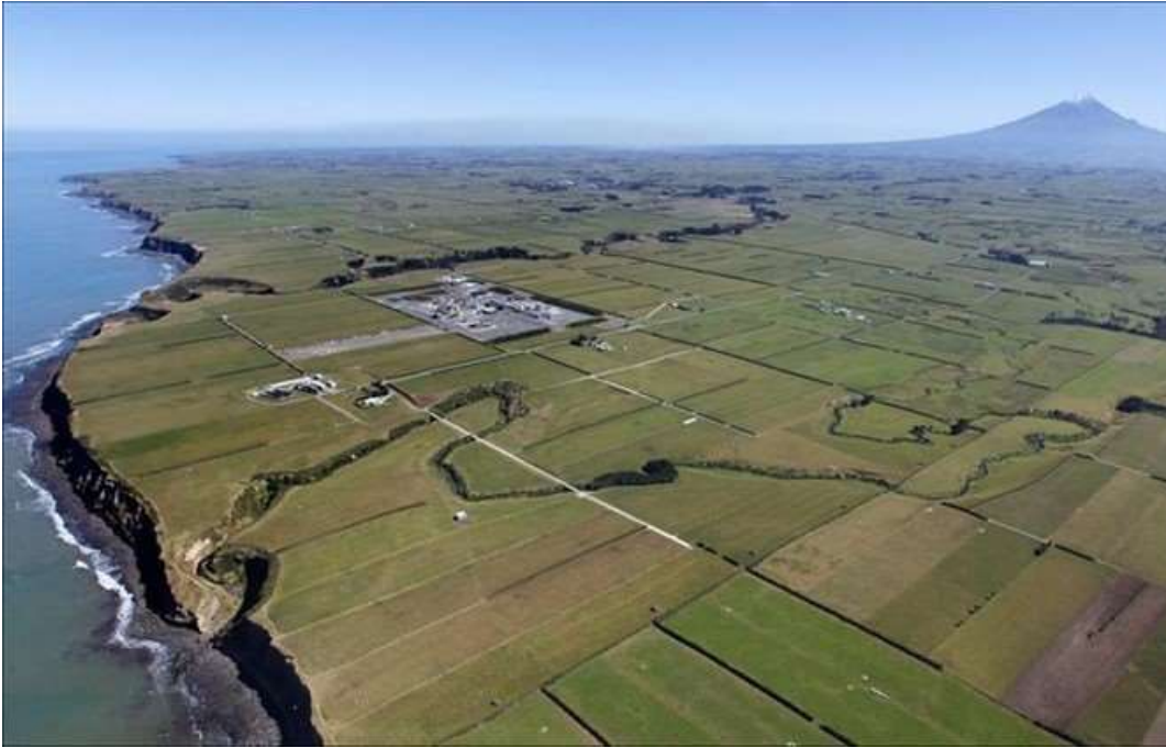
Photo 1 Kupe Production Station
