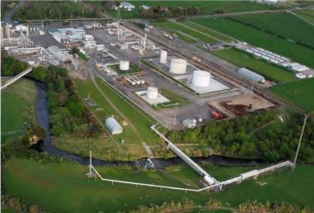
Photo 1 Kapuni Production Station
