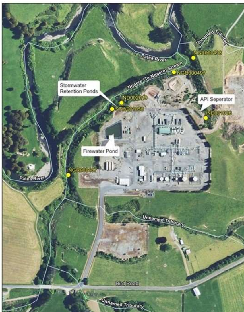
Figure 2 Waihapa Production Station stormwater systems and monitoring sites
