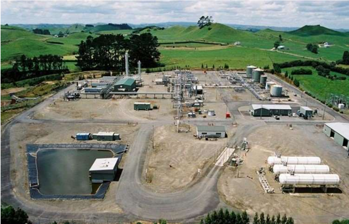
Figure 1 Waihapa Production Station
