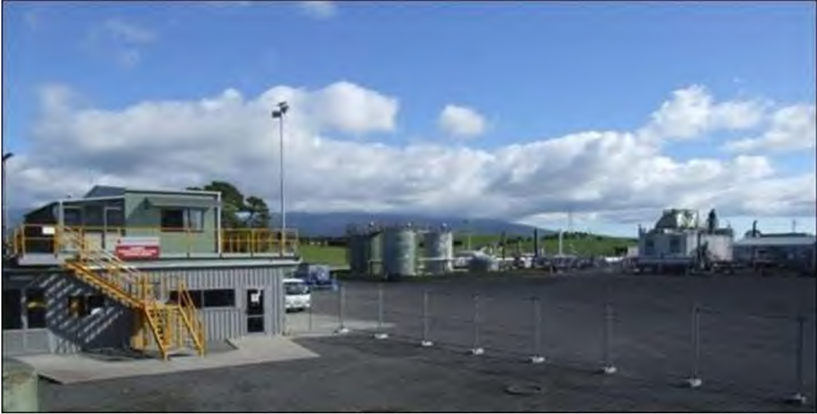
Photo 1 Kaimiro Production Station
