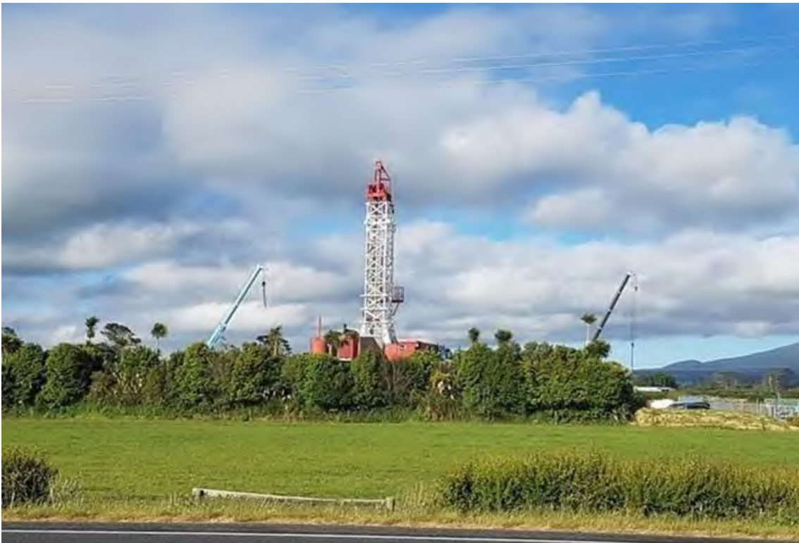
Photo 2 Radnor Production Station
