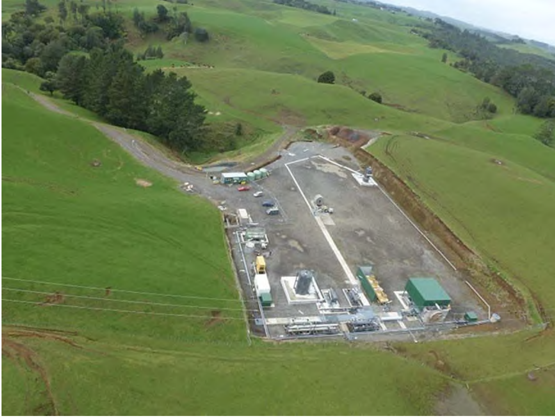
Photo 2 Kowhai-A Production Station
