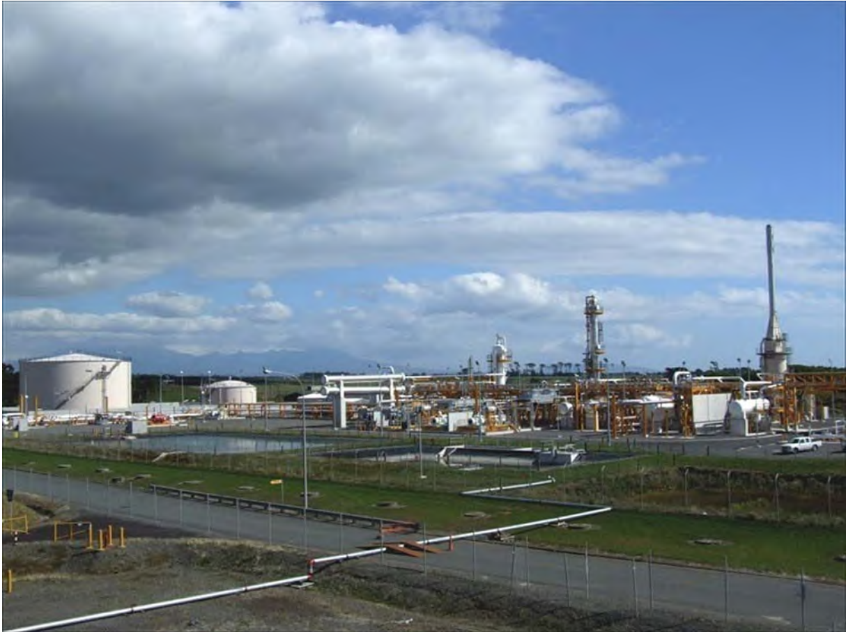
Photo 1 Pohokura Production Station
