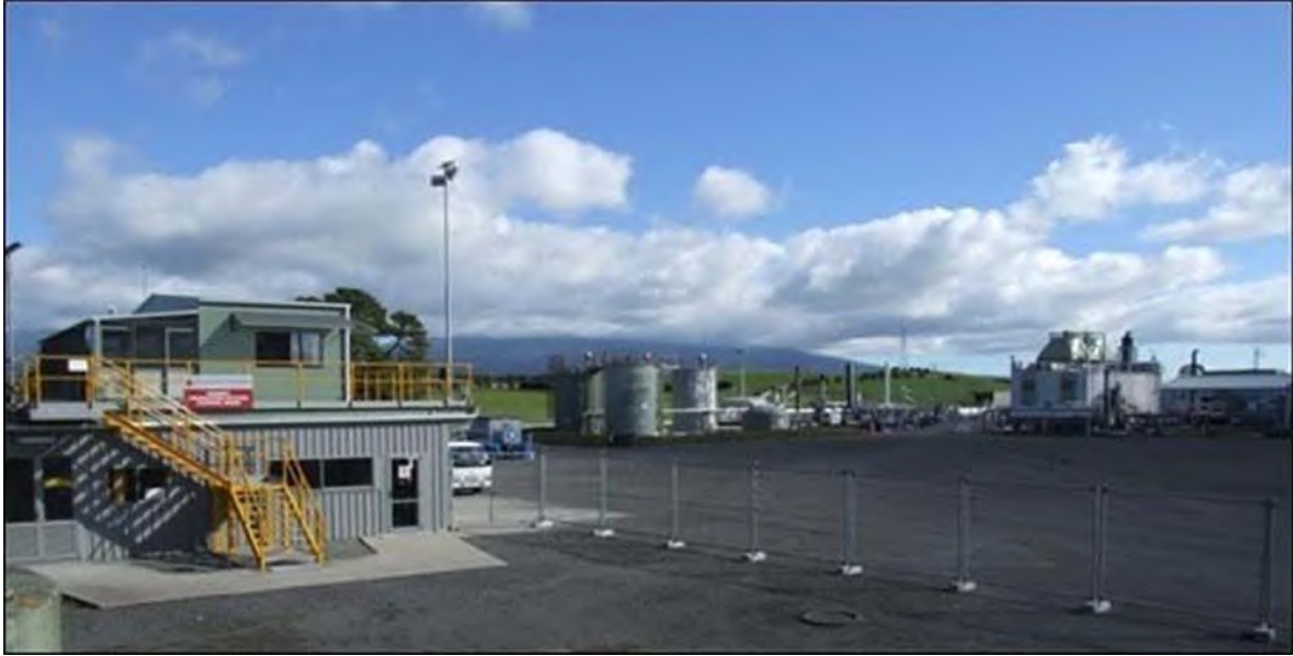
Photo 1 Kaimiro Production Station
