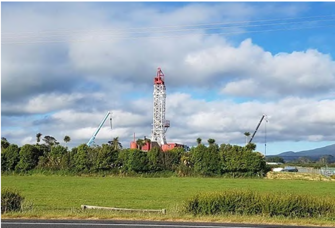
Photo 2 Radnor Production Station
