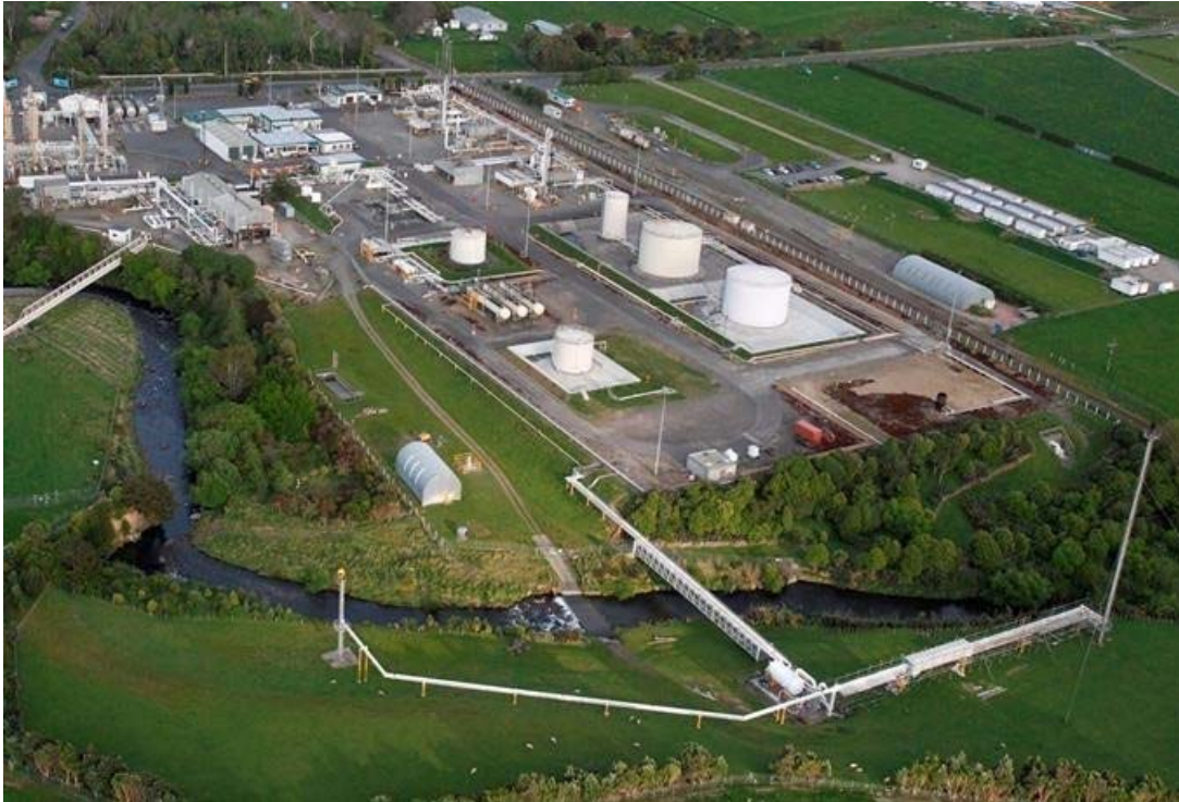
Photo 1 Kapuni Production Station
