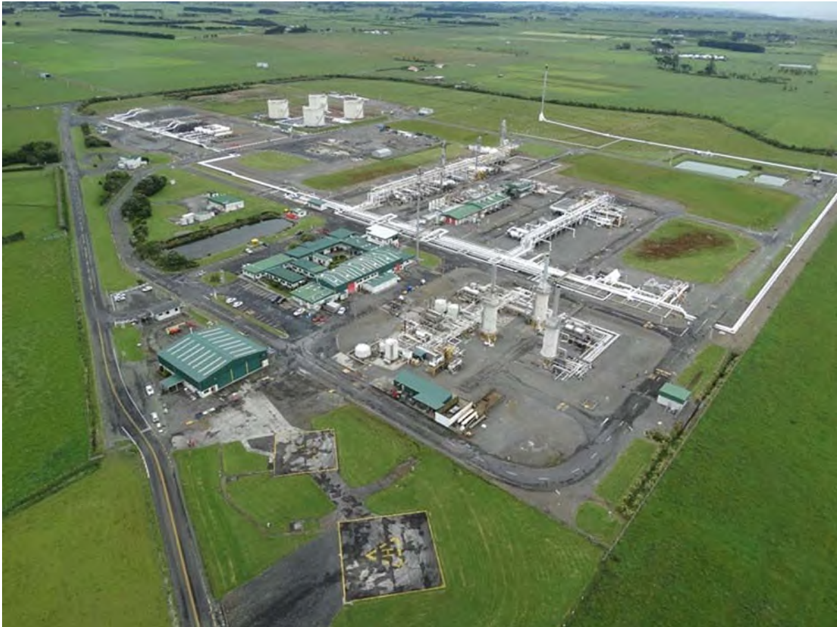
Photo 1 Maui Production Station
