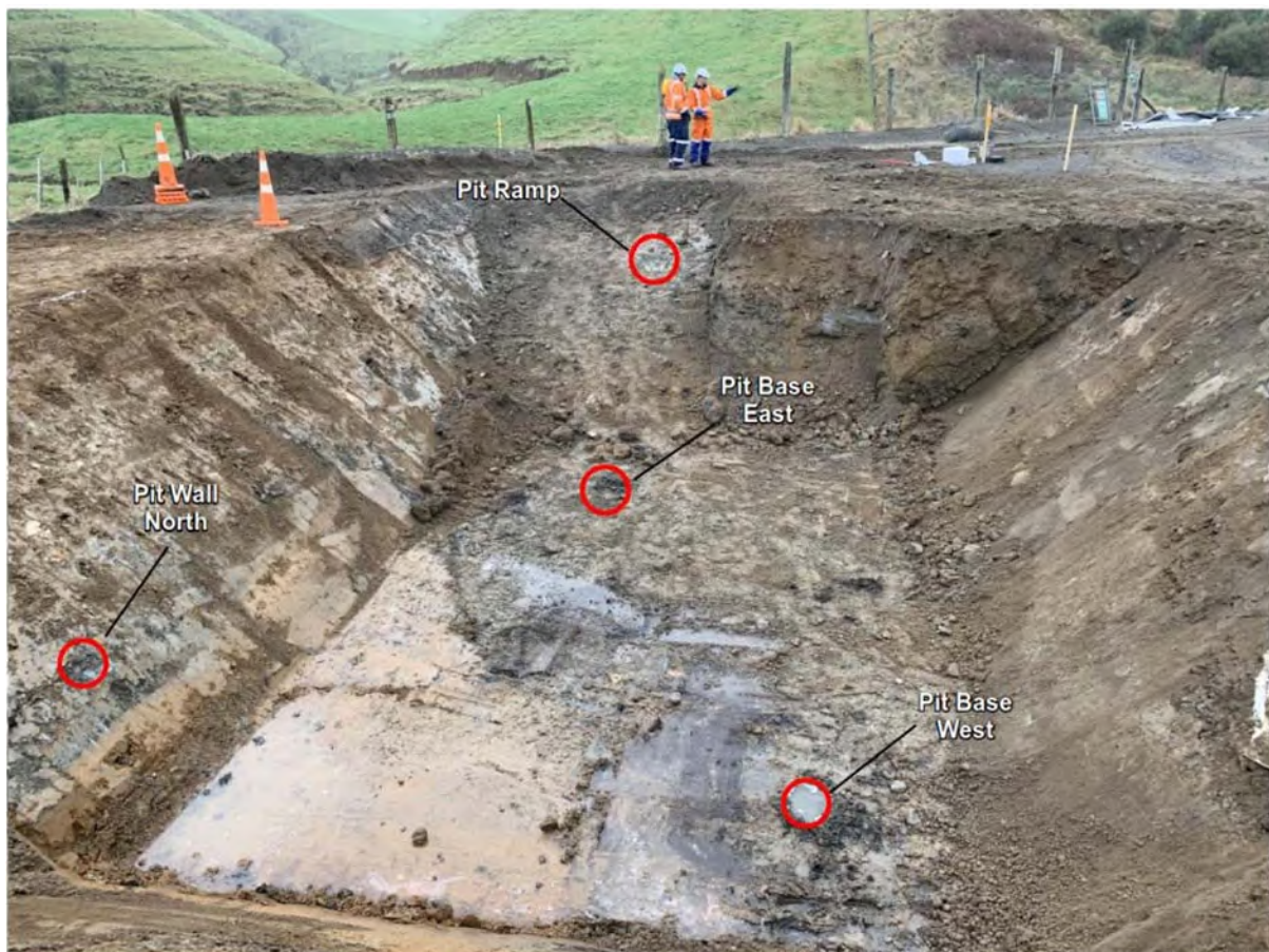
Photo 3 MBC consent 5173-2 and the new skimmer pit excavation sample locations
